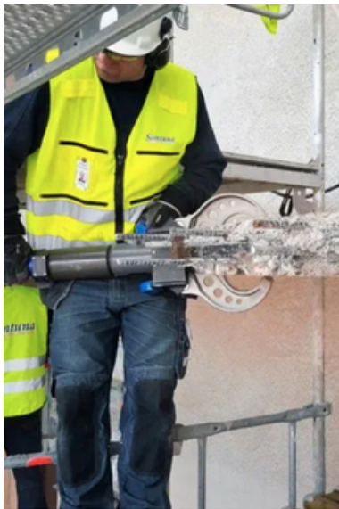
Img.1.2 Using handheld concrete crusher Source: Tehma SA 2
