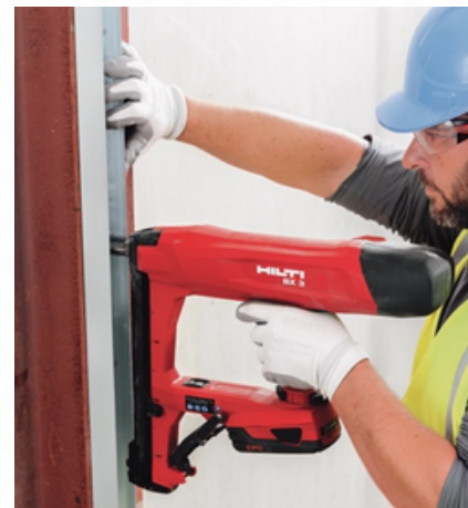
Img 2.5 Using battery actuated direct fastening machine Source: Hilti 5
