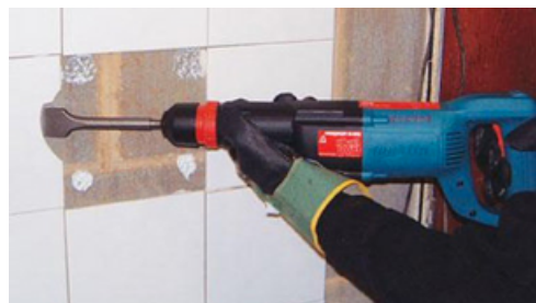
Img2.3 Using light-weight breaker Source: National Tool Hire Shops
