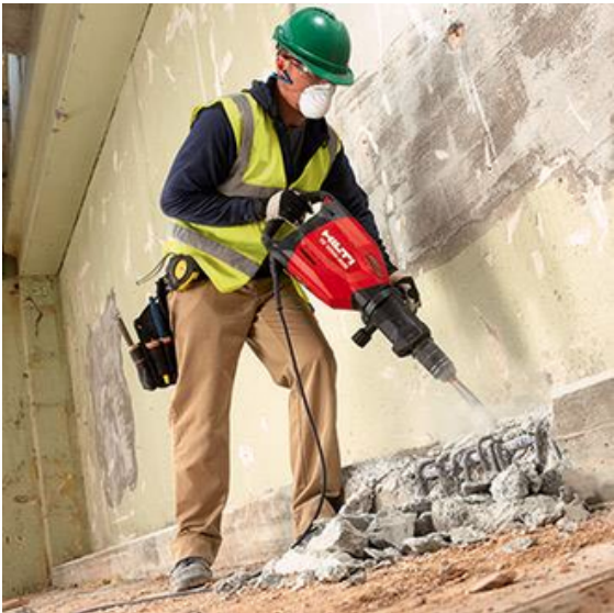
Img. 1.1 Using handheld breaker Source: Hilti 1
